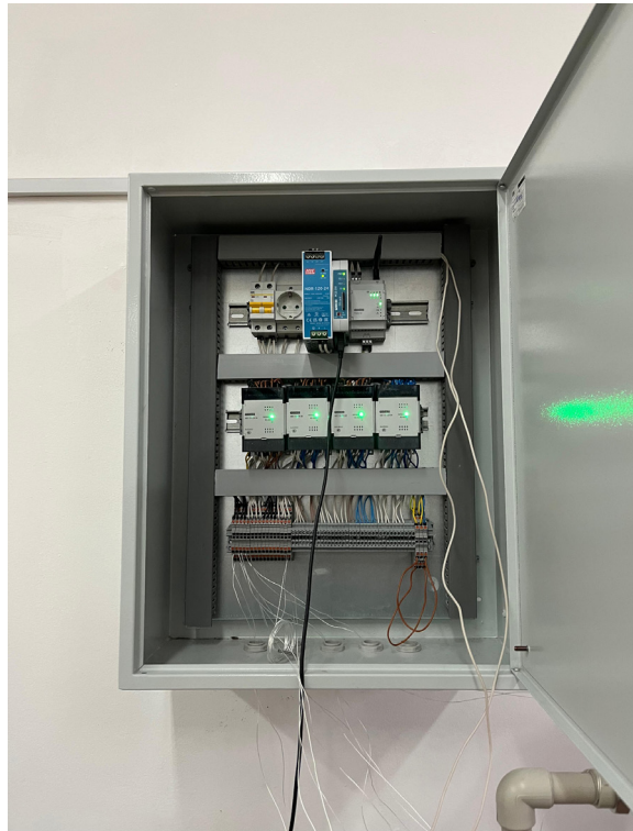
Figure 5 – Data acquisition layer
